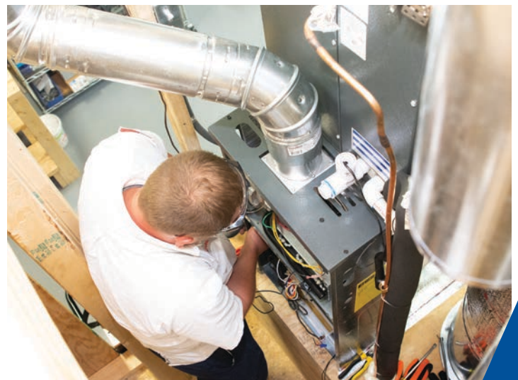
Student installing a new gas furnace and doing final checks.
